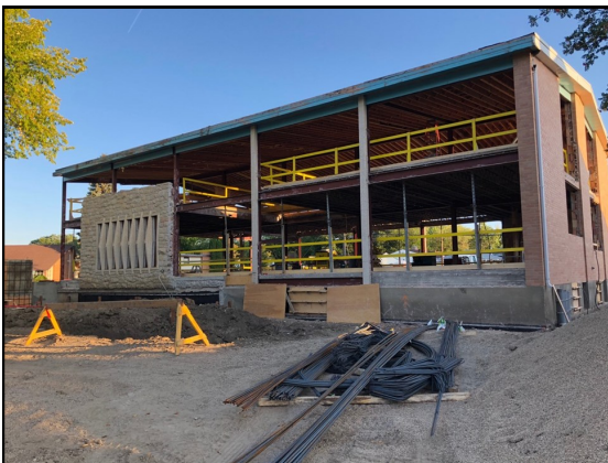
Front view of the original building being renovated.
