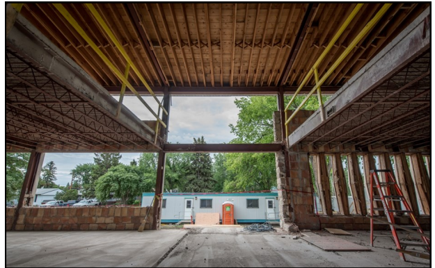
Renovation of the existing building, future foyer of the Hospice.
